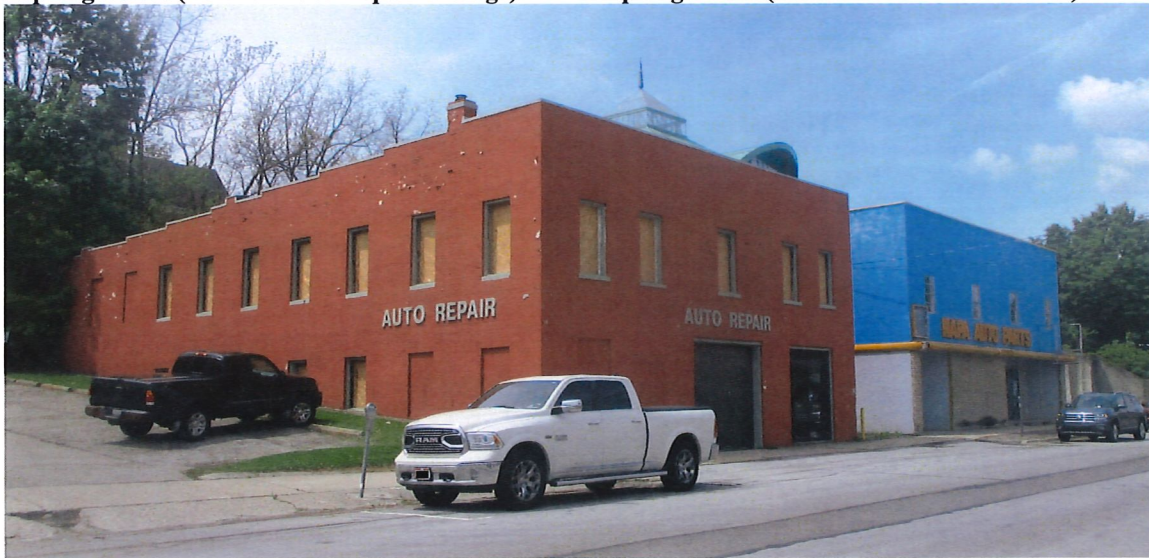
7 Spring Street (Former Auto Repair Garage) and 27 Spring Street (Former NAPA Auto Parts) – 2021
