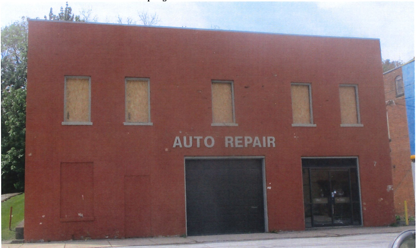
7 Spring Street – North Elevation - 2021
