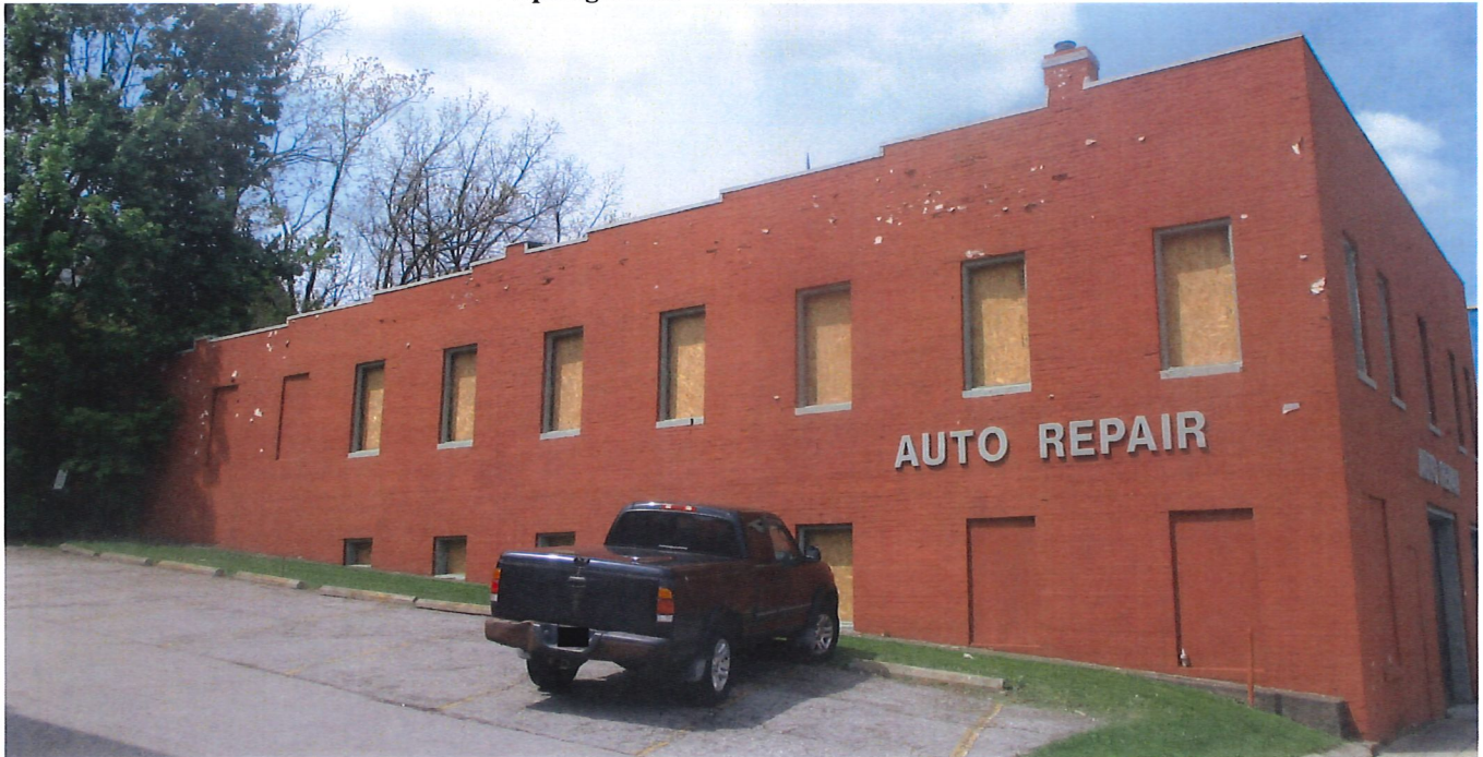
7 Spring Street – East Elevation - 2021
