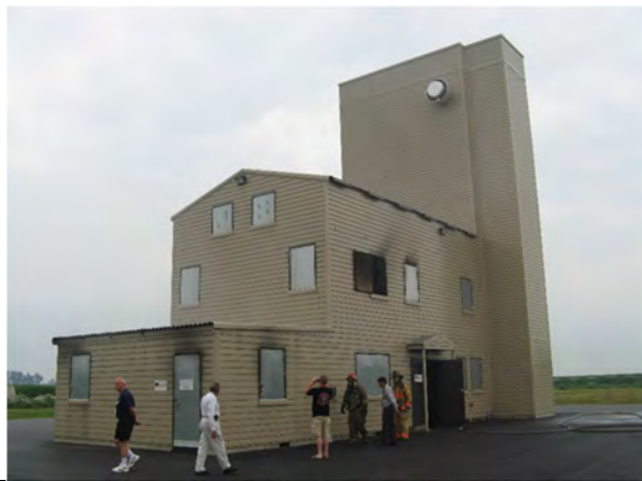
This is an example of a combination commercial and residential multi story training tower with live fire capabilities.
