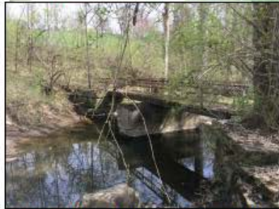
EXISTING BRIDGE NEAR GRADY MEMORIAL HOSPITAL
