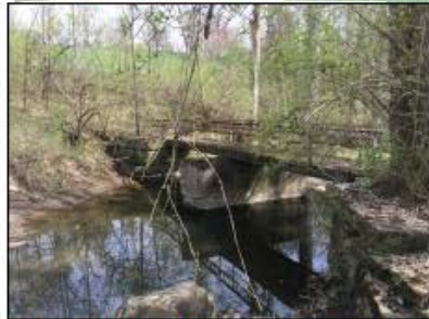
EXISTING BRIDGE NEAR GRADY MEMORIAL HOSPITAL
