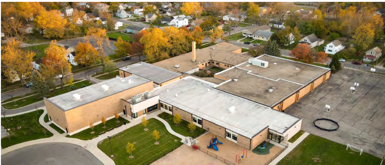
Woodward Elementary School provides a civic anchor in the center of the neighborhood
