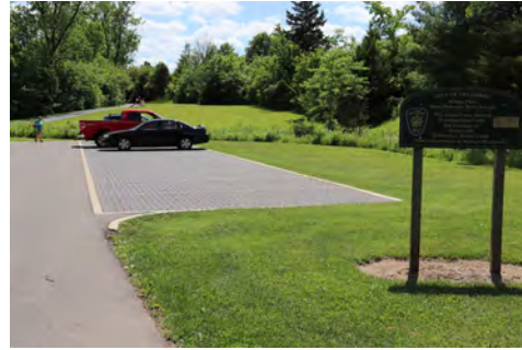
The City has used permeable pavers in parks, in ways that can be a model for private developers.
