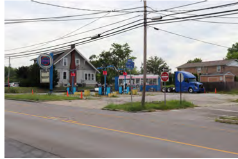
Sites such as old gas stations are ideal candidates for remediation.
