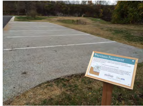
Permeable pavement has been installed at Blue Limestone Park helps to manage stormwater and provide numerous environmental benefits.
