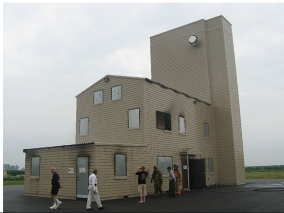
This is an example of a combination commercial and residential multi story training tower with live fire capabilities.
