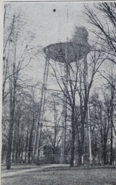
SENTINEL OF SAFETY — Located in the city park in the block bounded by Liberty, University, Washington and Park Streets, the 250,000 elevated storage tank shown in the picture is the basic reserve supply of water for the city. A 250,000 open, standpipe near the waterworks has been ordered rehabilitated or removed by the state health department. Replacement of the standpipe by a 500,000 elevated storage tank within the city limits is contemplated for 1956 or 1957. During 1955, the average daily consumption of water in the city was approximately 1,200,000 gallons.
