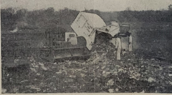
AFTER NEW SYSTEM — Sanitary Fill Reclaims Low-lying Property — One of the city's packer-type garbage and rubbish collection trucks unloads. Also shown is the city's crawler tractor with bullecan attachment which spreads, compacts and covers the material continuously. As well as eliminating the rat and odor problem and minimizing the fly problem, this method of refuse disposal makes possible the reclaiming
