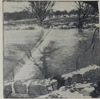
COMPLETED LOW DAM — Here is the lower Olentangy River dam to be completed this spring. The pool immediately to the north is three feet deep and the water then feathers out toward the upper dam between E. Central and E. Winter Sts. Both dams were built with money raised through a voted bond issue and a $13,000 additional amount granted by city council. The lower dam is south of the New York Central bridge and north of Hayes St.
