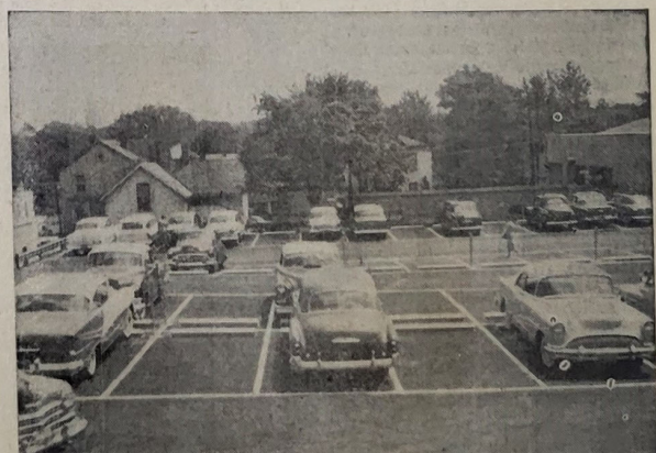
E. WINTER STREET PARKING LOT SELF-SUPPORTING — This is a typical scene at the city's first parking lot on E. Winter Street. Originally designed for 84 cars but subsequently altered to 65 cars due to widening of stalls, this lot is producing more
