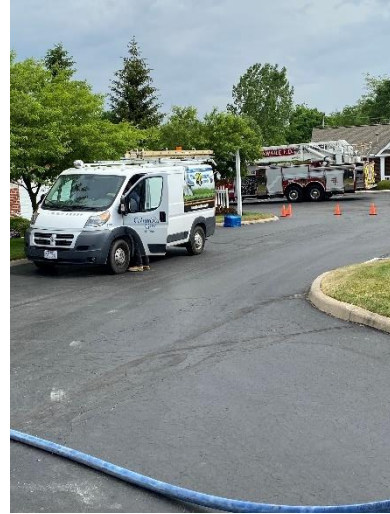
May 26 – Natural Gas Leak
