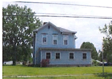
Renovating older homes helps preserve the character of existing neighborhoods while advancing fiscal and economic sustainability goals.
