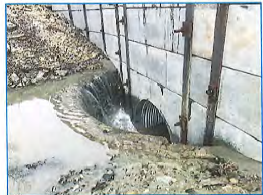
New spillway and culvert along Sugar Run
