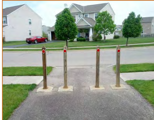
Figure 3-7: At this location off Timbersmith Drive, bollards nearly prevent bikes from entering/leaving the roadway, forcing bicyclists (and those using a wheelchair or stroller) to leave the path.
