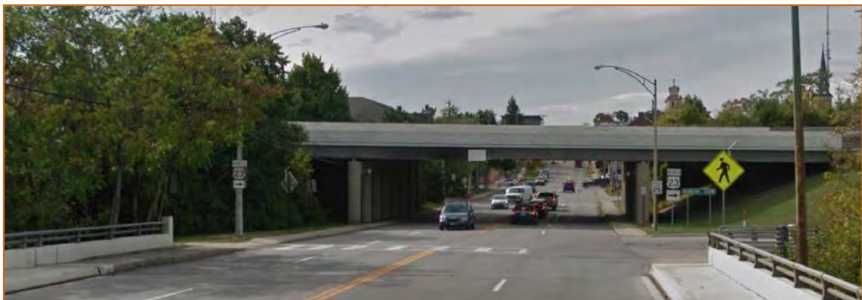
Figure 3-6: Mingo Multi-use Path at its crossing of SR-37 looking south. While the crossing has continuously-flashing beacons and is striped, a median island, pedestrian-activated push button, and a wider and more direct north approach would improve accessibility and safety for all users.
