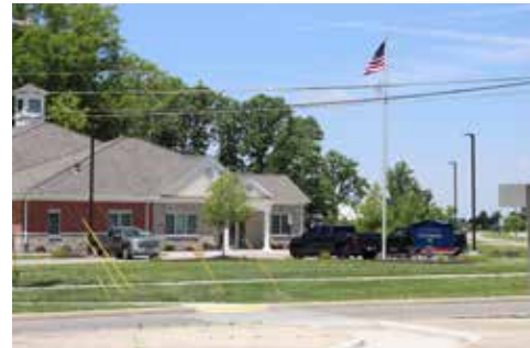
Fire Station 304 was completed in 2019 at Cheshire Road and Glenn Parkway designed to increase public safety in the southeast corner of the City, where the population has grown to more than 5,000 residents.
