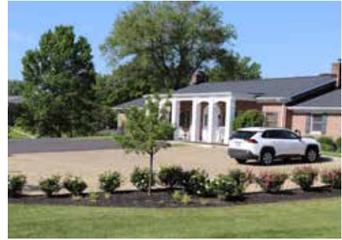
An eco-paver used at an assisted living facility is an example of a permeable surface that can help with stormwater management.
