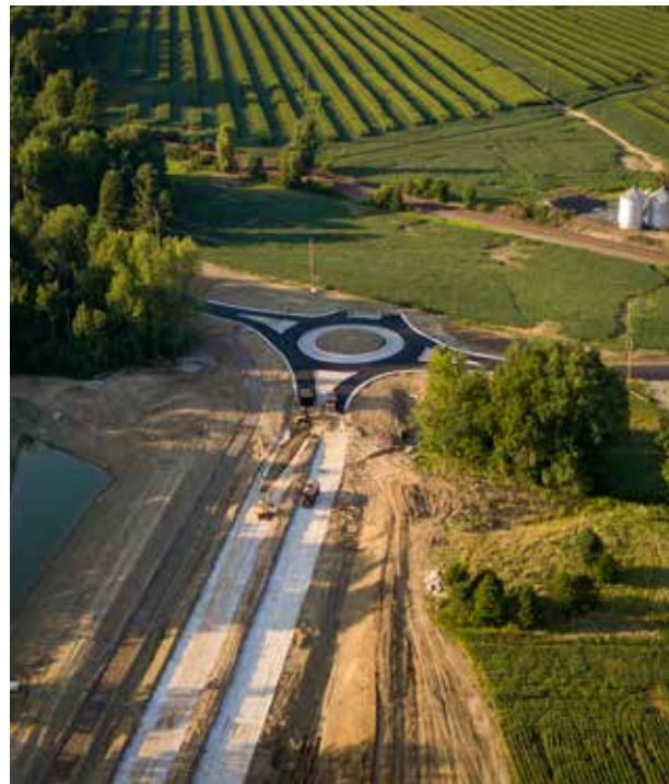
View of Glenn Parkway at Berlin Station Road, which has been completed.
