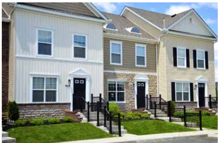
Multifamily, rental housing that functions like single family attached housing developed at Carson Farms (above) has provided a housing alternative for those seeking lower maintenance option.
