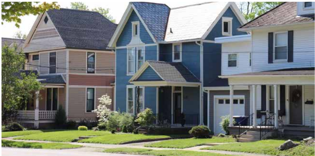
The City has prioritized historic preservation, retention of existing character, and sensitive infill development in traditional neighborhoods.
