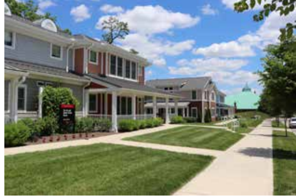
Ohio Wesleyan University's Ditttrick House is a redevelopment project that provides duplex-style small living units (SLUs) for students.
