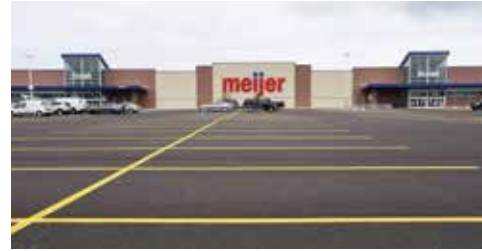
Over-parking can increase vehicle trips unnecessarily and should be avoided when possible.
