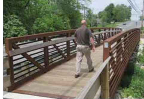
High quality pedestrian connections make travel by foot more convenient, safe and enjoyable.
