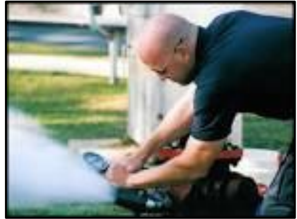
Public Utilities conducts maintenance on fire hydrants
